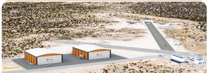
Tech1 Campus-Bravo Site Tornillo, TX
