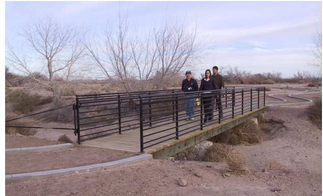
The new footbridge on the Bosque Trail.
