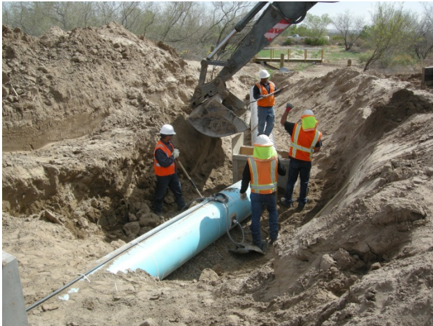
El Paso County Water Improvement District No. 1 personnel install turnout from Riverside Canal to Rio Bosque, April 10, 2013.
