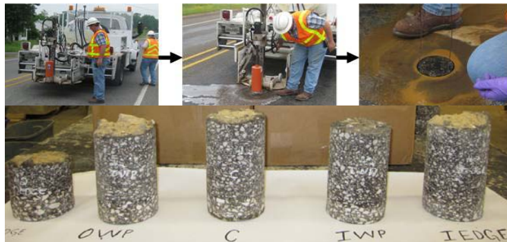
Figure 8.3 - Coring operation for a Core Profile across a Pavement Section.
