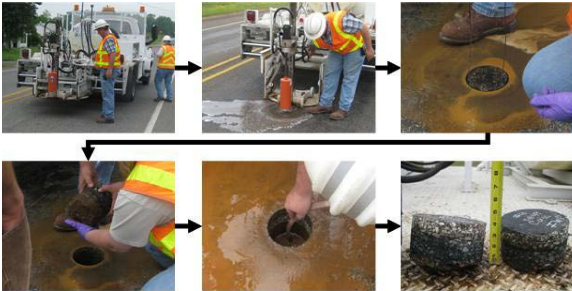
Figure 5.9 - Coring Process Images.
