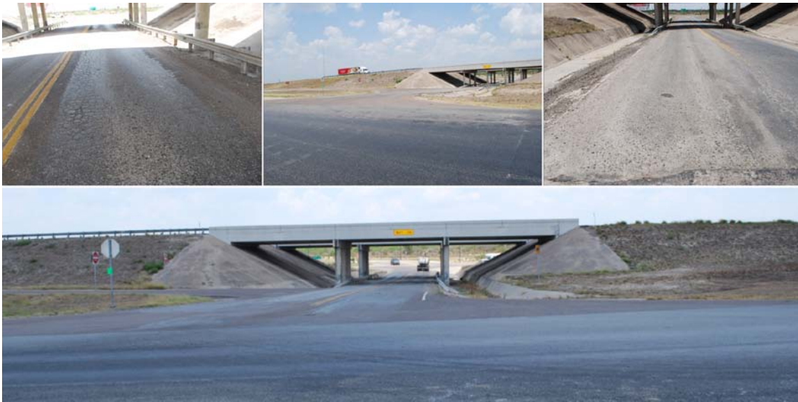
Figure 7.13 – Views of Conditions of US 83 and I-35 Intersection.
