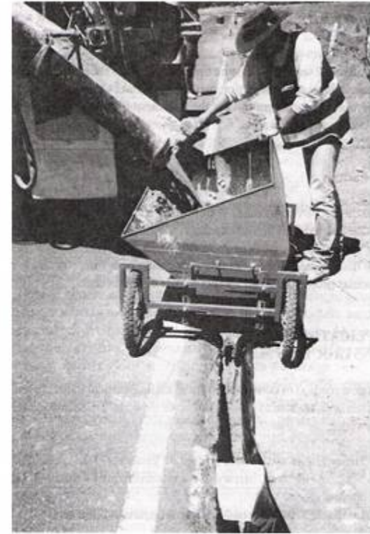
Figure 5.5c - Membrane, Polystyrene Wedges, and Placement of Flowable Fill
