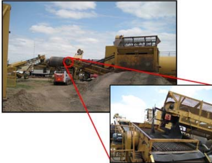
Figure 2.1 – Screening Unit Used to Prevent Large RAP Particles from Entering Mixture
