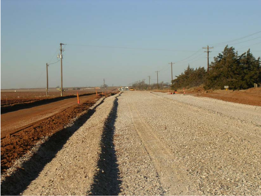
Figure 5.2 – Addition of Add Rock
