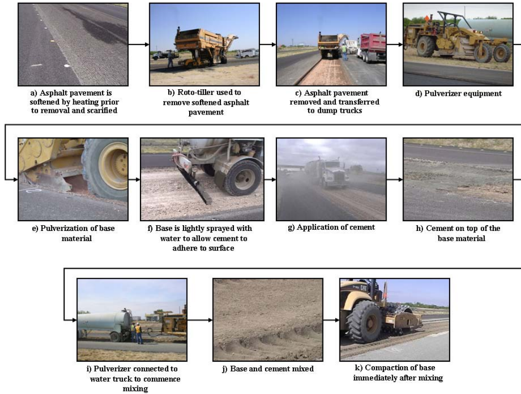
Figure 4.1 – Construction Procedure used for I-10, and I-20
