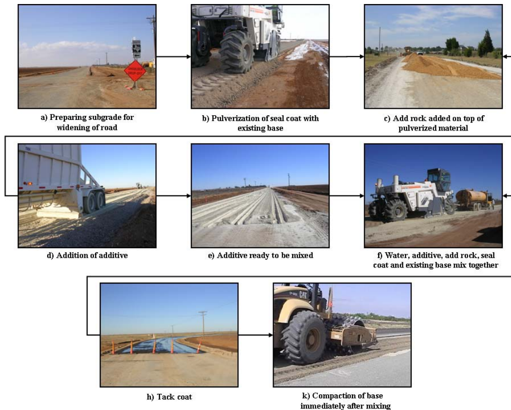
Figure 4.2 - Construction Procedure used for FM 1939, FM 303 and FM 905
