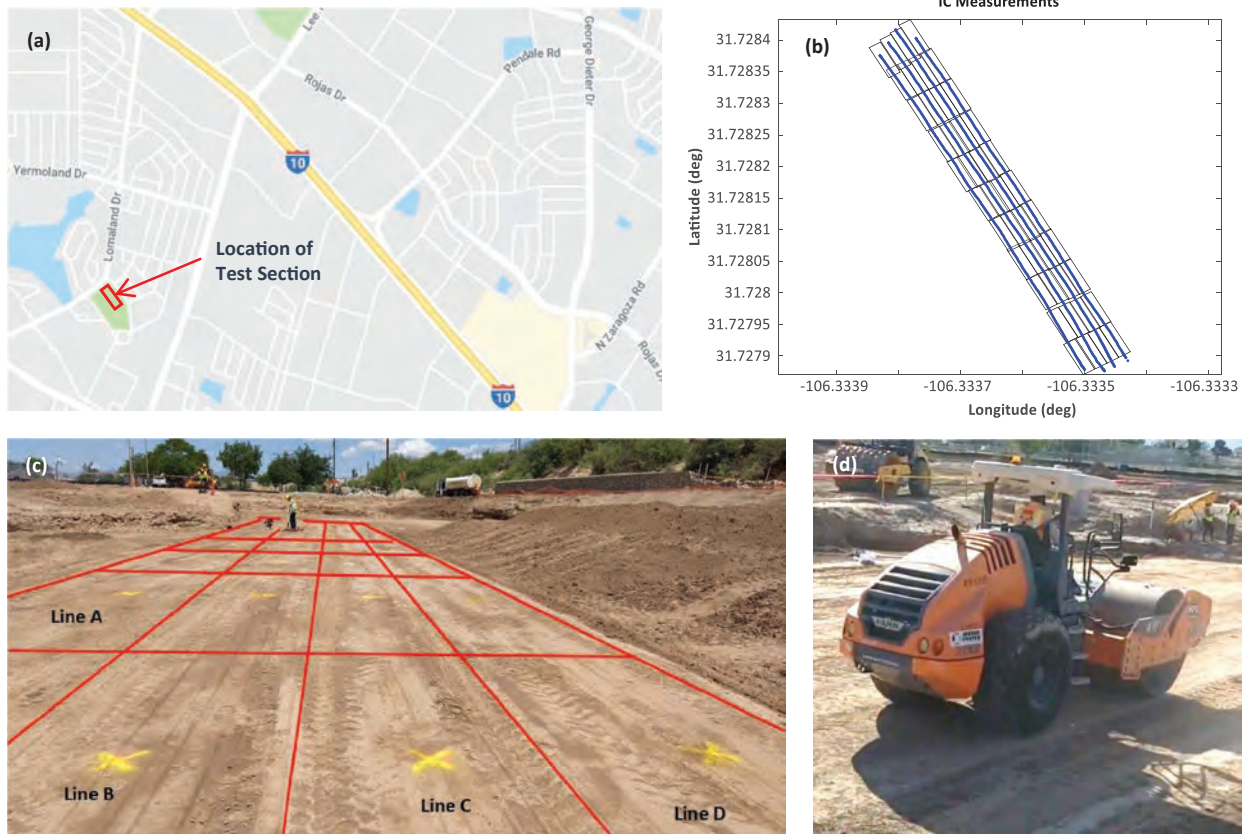
Figure 7-2. Overview of Lomaland Recreational Center construction in El Paso, Texas, showing (a) location of test site, (b) line passes during proof mapping of embankment, (c) test section with sublots, and (d) IC roller used at this location.
