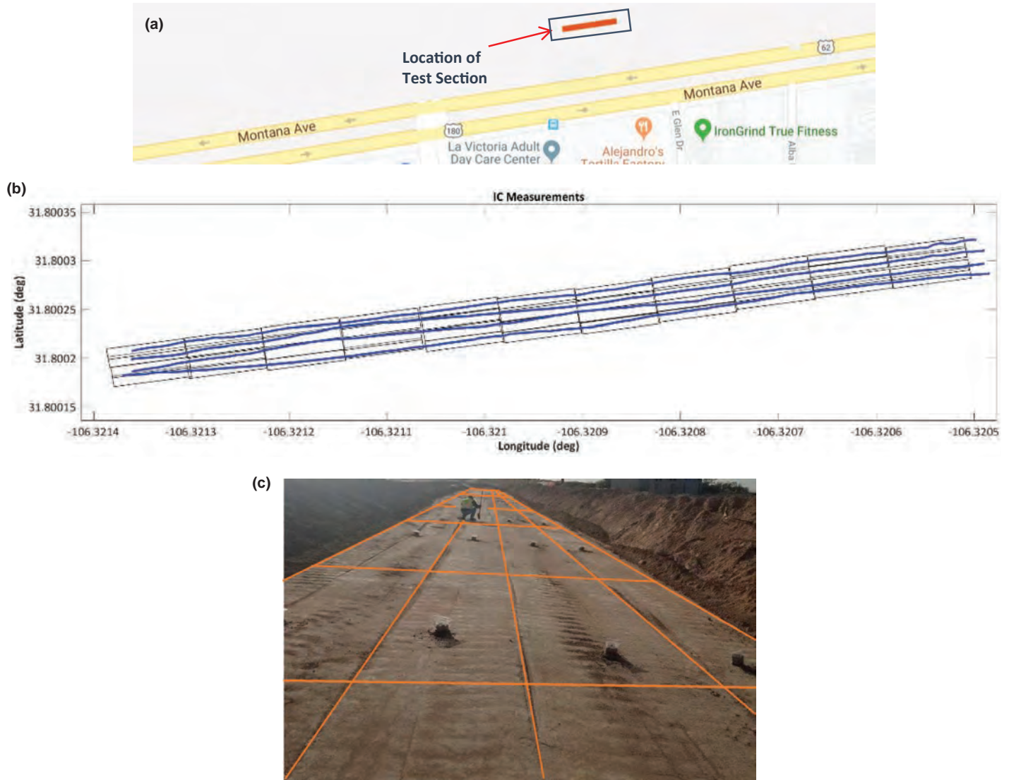
Figure 7-5. Overview of US-62/180 westbound construction of Montana Expressway in El Paso, Texas, showing (a) location of test site, (b) line passes during proof mapping of subgrade, and (c) test section with sublots.
