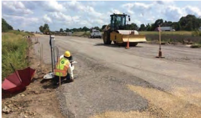
Figure 4-7. UTEP personnel monitoring proof-mapping process.
