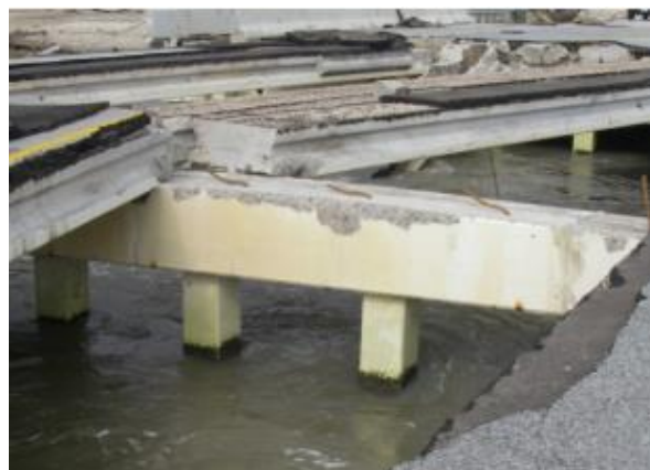
Figure 17. State Highway 87 Rollover Pass Bridge along the Texas Coast [28]
