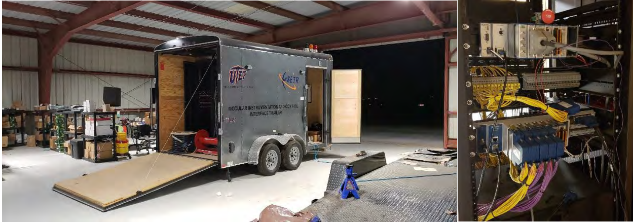
Figure 1: (left) Outside view of the MICIT trailer (right) wired compactRIO and compactDAQ
