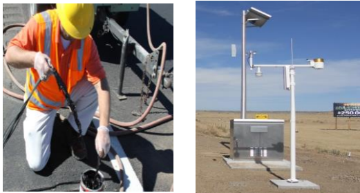
Fig. 1. Installation of temperature probes and weather station.
