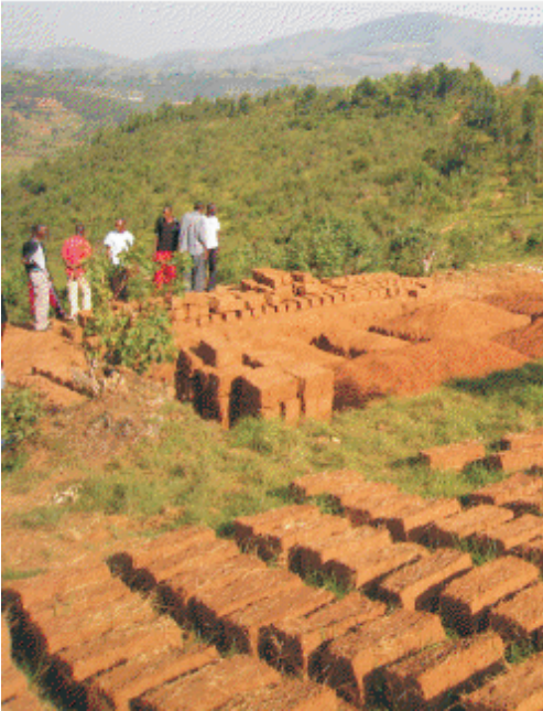
Typical village building site, 2009
